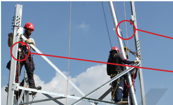
Figure 5 – New TVL system, indicating the position and the purpose of the TVL.
