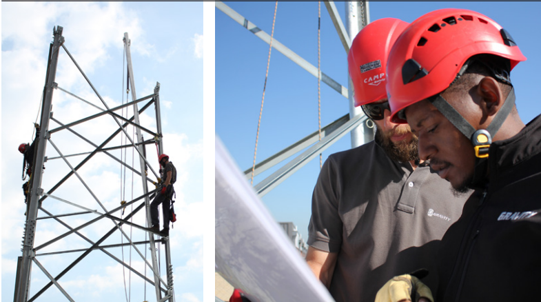
Figure 1 & 2 – Typical scenarios depicted when erecting towers.
