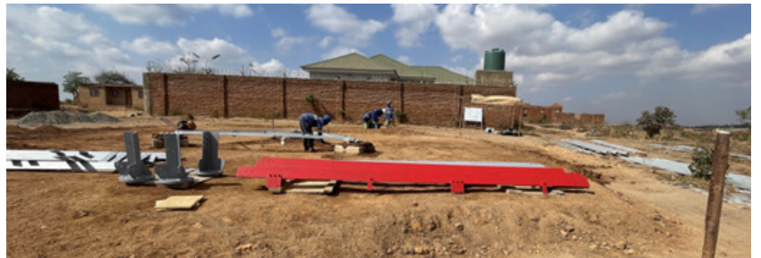
Figure 6 – Typical site layout before the erection of the tower starts.
